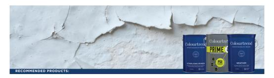
Peeling or flaking paint on concrete can be the result of two issues, it can be due to moisture being trapped under the paint or it can be a result of the paint not adhering to the substrate. To prevent this issue recurring the source of the problem must be identified and treated prior to repainting.
