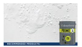
Blistering paint is identified as small bubbles or blisters under the paint layer. The causes and treatment of blistering paint are similar to flaking/peeling paint. There are many reasons for blistering paint on all surfaces.
